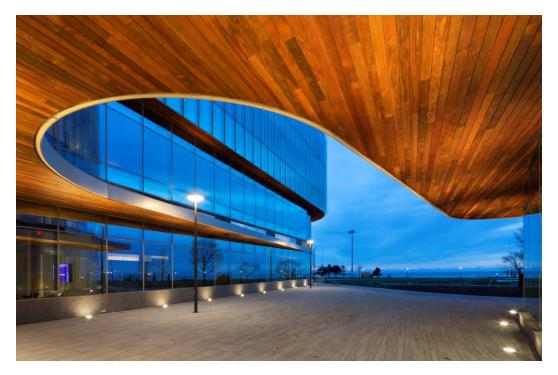
The Kellogg Global Hub design team's solution was to use an innovative system to attach the wood soffit: the Iron Woods® Vanish™ Rain Screen and Soffit System.
