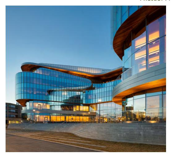
The Iron Woods Rain Screen and Soffit System is an engineered system in which all of the design components play an interdependent role in the system's performance. Each installed system is stamped and certified by a licensed state engineer to comply with state building code wind load compliance requirements.
