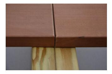
Taking it one step further we have also seen contractors use biscuits or dowels to eliminate any potential for movement at the butt joints. When using hidden fasteners with or without biscuits or dowels double up the clips at but joints to make sure a mechanical connection is achieved between both pieces of decking to the stringers to maintain consistent gapping and prevent shifting as shown below.
