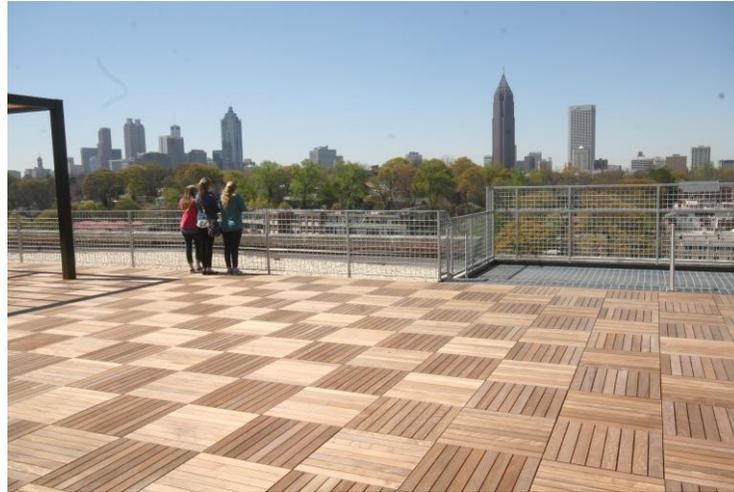
Iron Woods® Elevations™ 24" x 24" Deck Tiles are a great option for conventionally constructed decks as well. Simply double your stringers 24" on center and fasten down at the corners with 4 Pro Plugs™ per tile. Iron Woods® deck tiles provide a unique appearance while at the same time significantly lowering overall construction costs. Deck tiles can be installed to create a wide range of designs and patterns.
